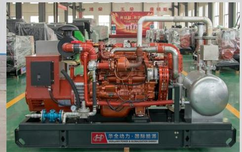
Its main equipment includes an engine, generator and heat recovery device. The working principle is that the biogas is supplied to the gas generator set by the storage tank through the desulfurizer, which drives the biogas internal combustion engine to generate electricity. The heat in the cooling water and exhaust gas discharged by the biogas generator unit can be recovered by the heat recovery device, and can be used as the heat source of the biogas generator.
